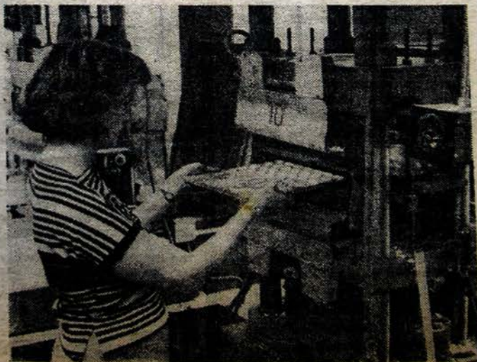
Future plastic earring buttons enter compression machine.
